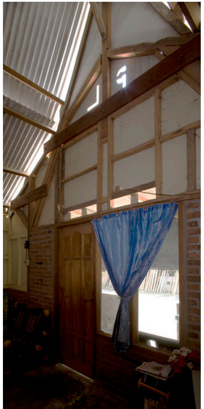
Interior view, with the panels on the wooden beams.
