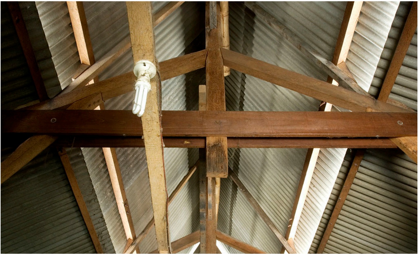
Detail of the wooden roof.
