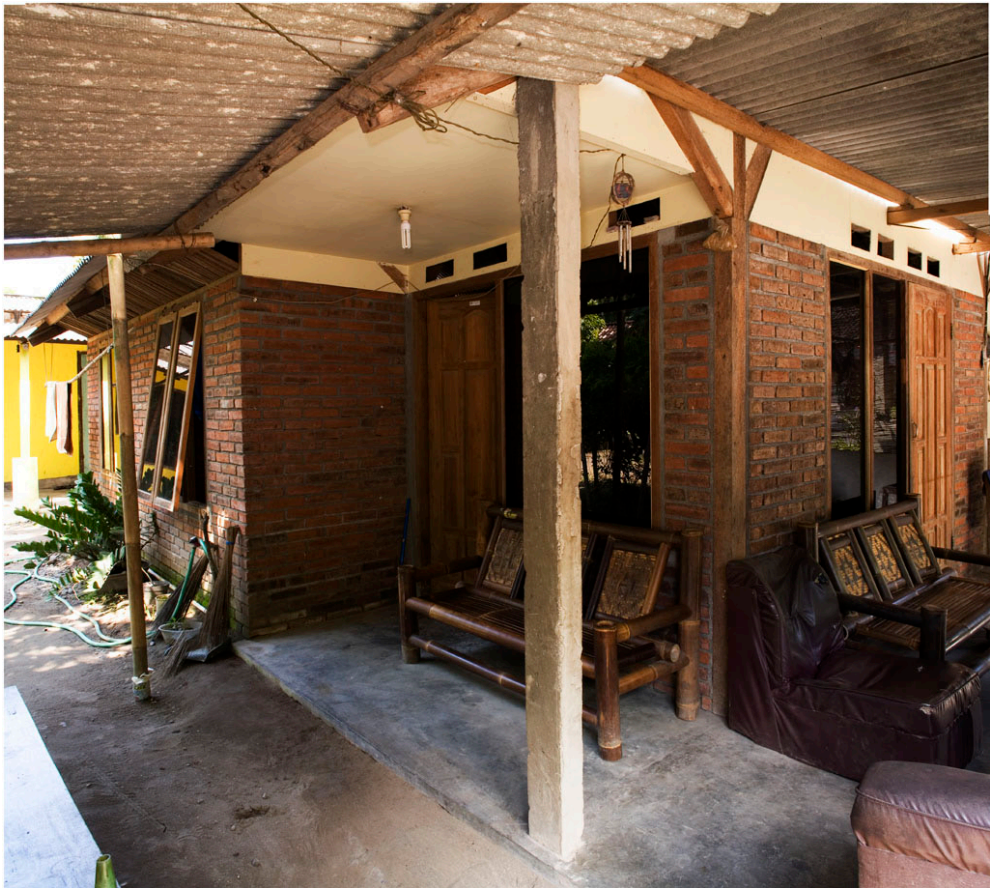
Terrace under the canopy roof, made of wooden beams and panels.
