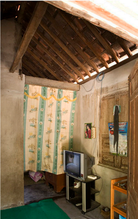
Living-room, and view on the wooden roof.
