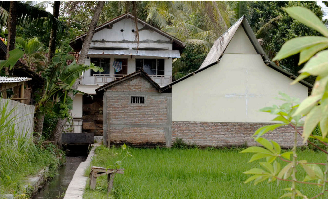
Rear view of a house made of brickwalls combined with fiber cement panels.
