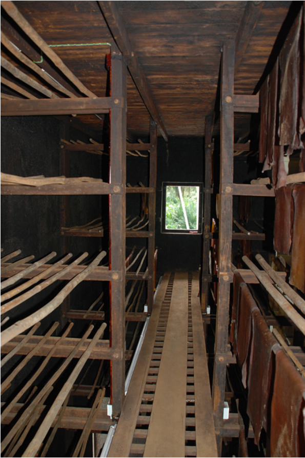
Smoking room before restoration.
