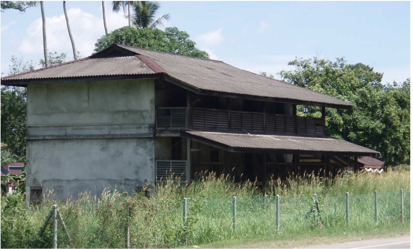
The Rubber Smokehouse before restoration.
