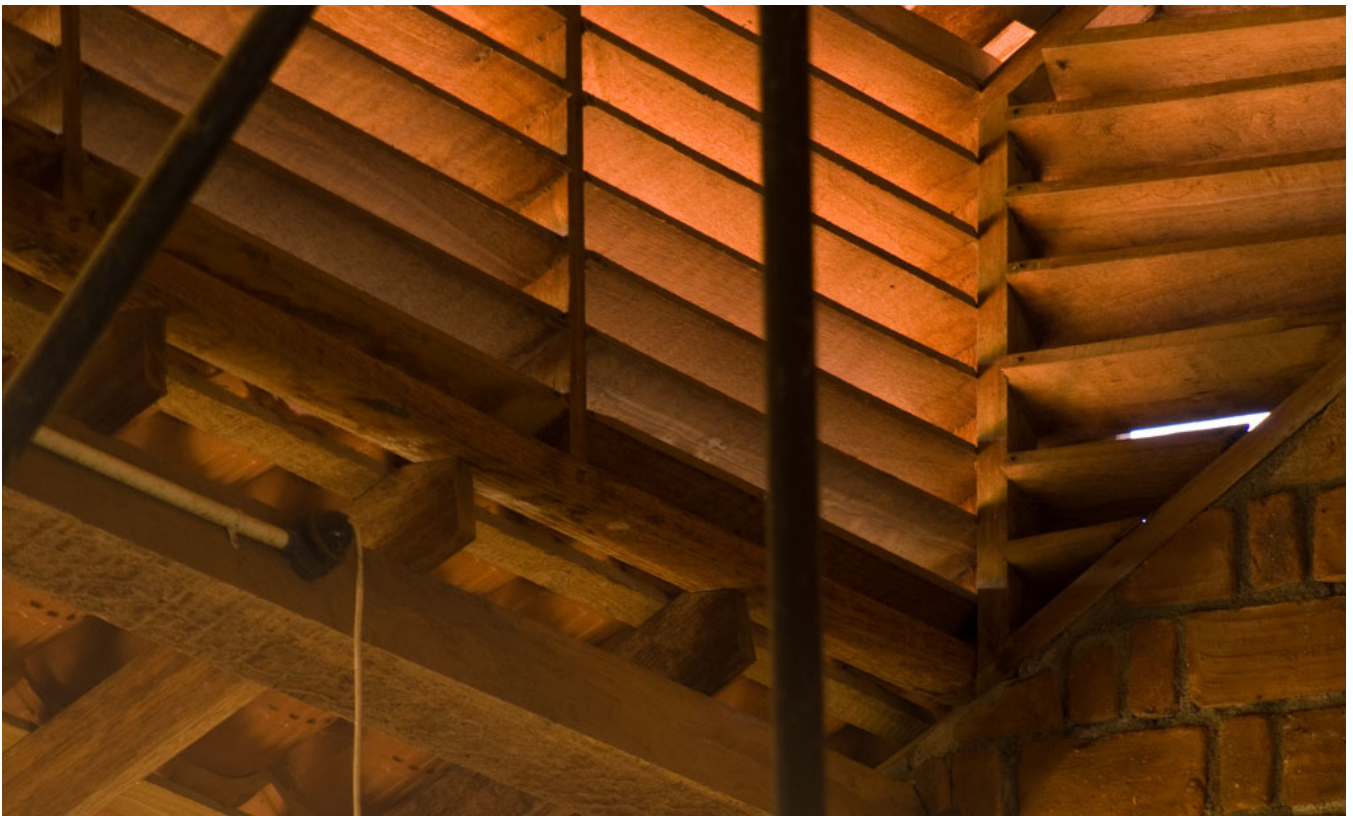
Detail of timber louvres in the computer room.
