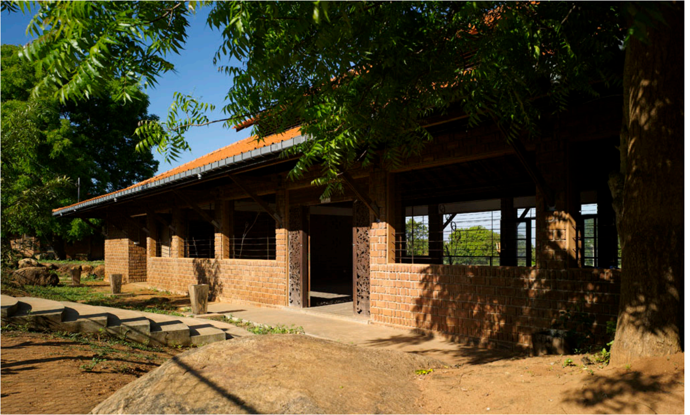
Entrance to the community building from the road.
