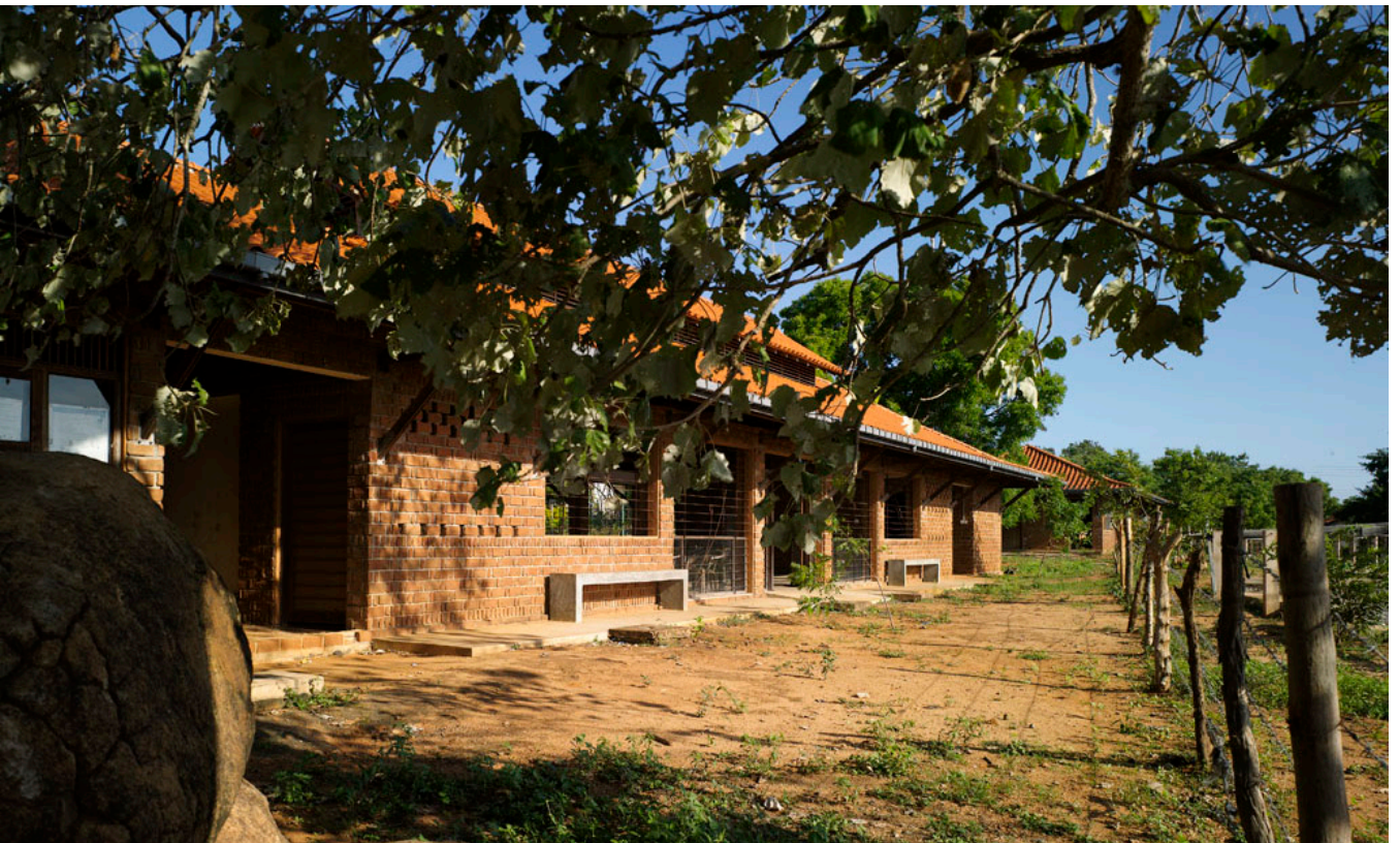
Rear view of the community building, facing the playground.
