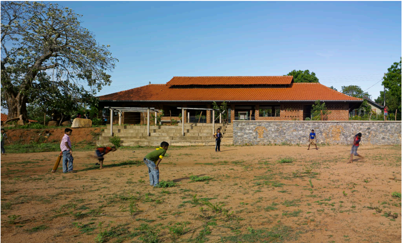
North -East view of the community building, from the playground.
