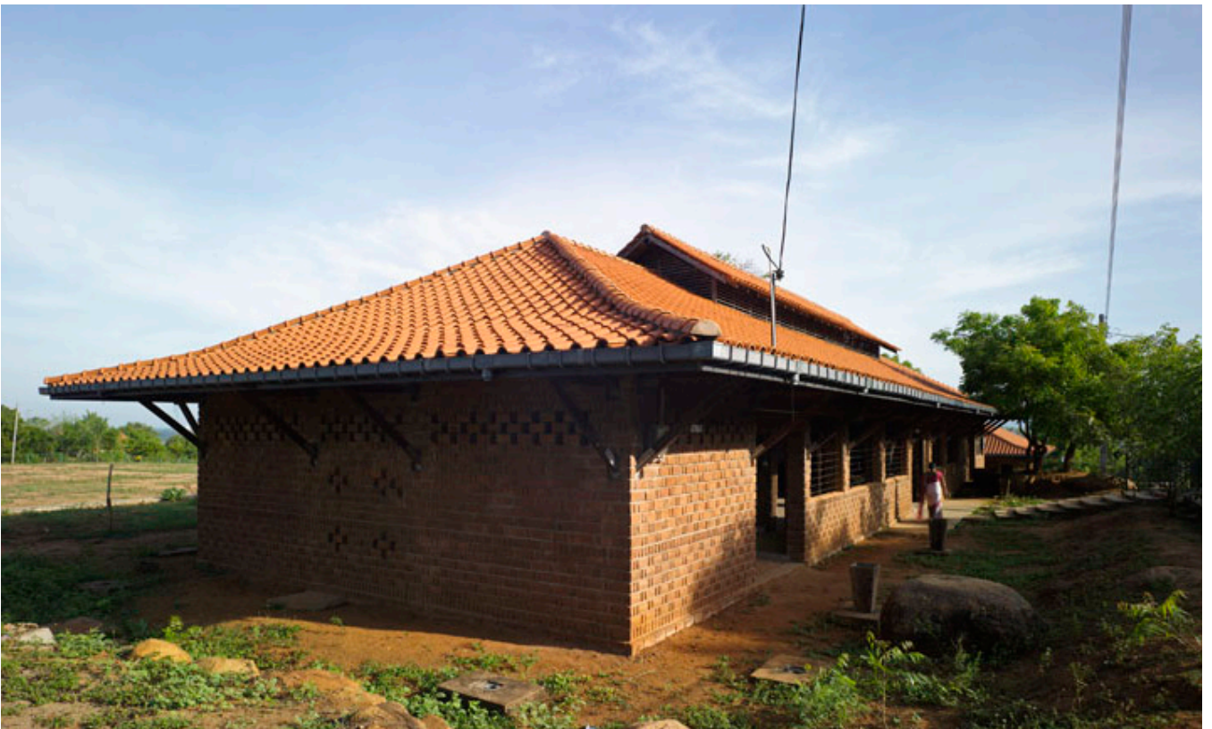
South view of the community building from the inner forecourt of the premises
