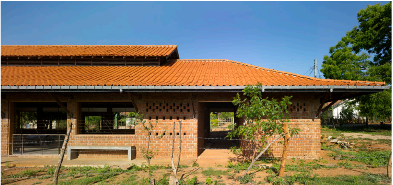
North-East view of the Community building.
