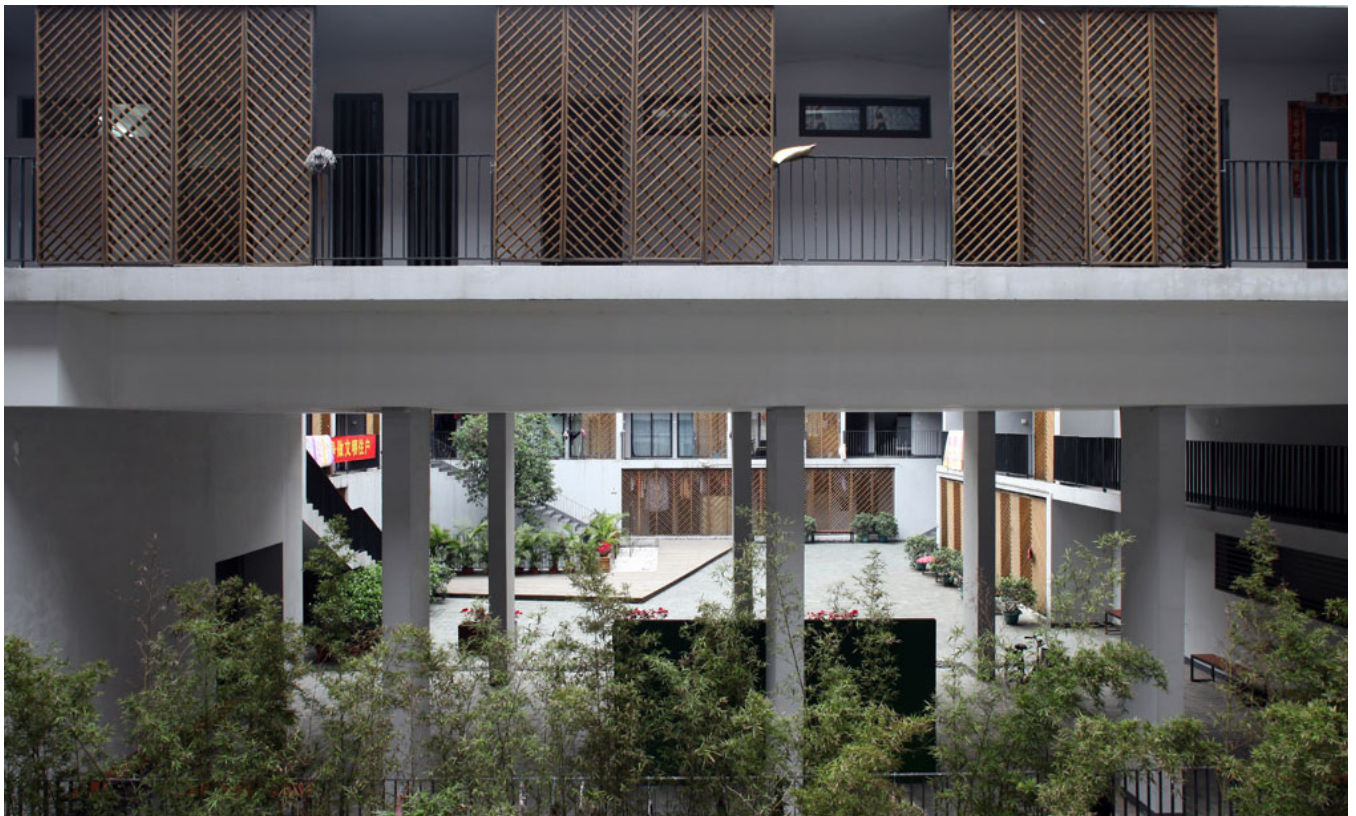
View of the central courtyard.
