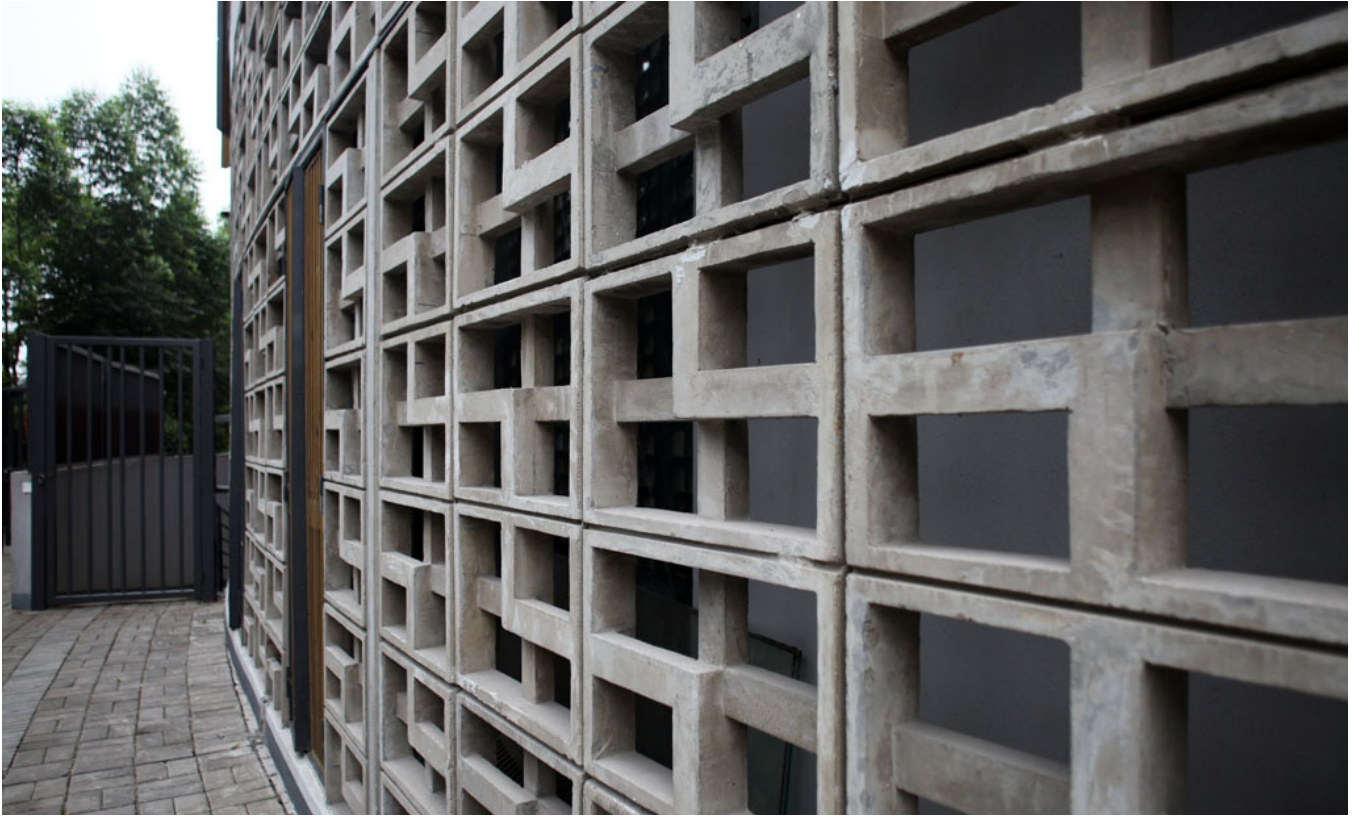
Detail of an exterior wall.
