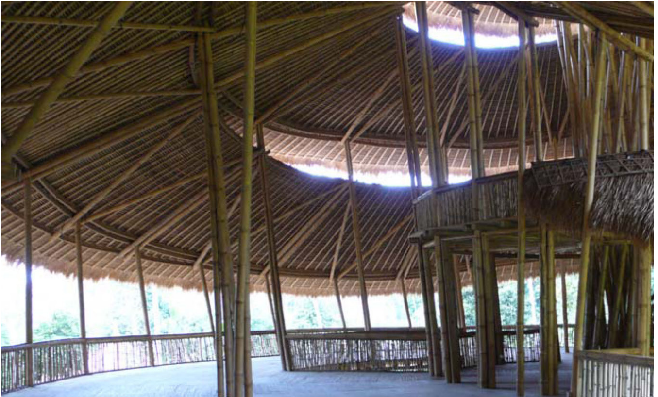
Interior view of the Heart of School bamboo roof.
