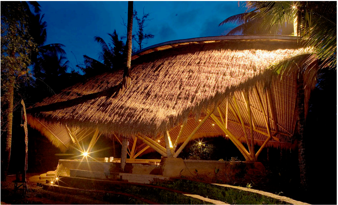
Megantigan studio, exterior, multifunctional school/community/performance space.
