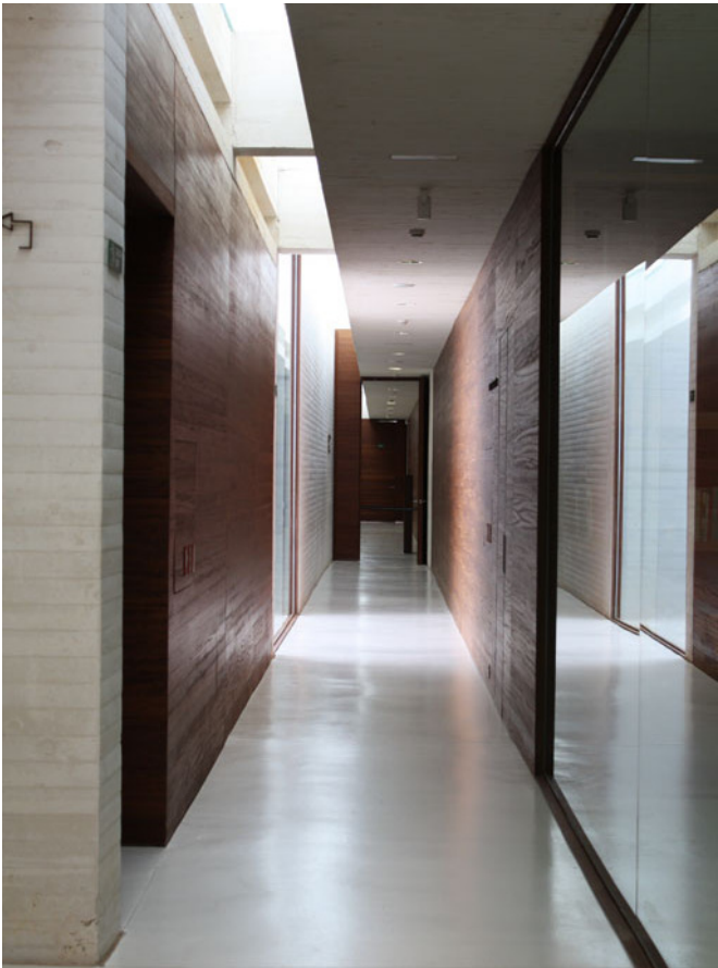
Corridor on the south side of the building. The white concrete is textured by the wood formwork - and the rhythm is repeated by oroko wood paneling.
