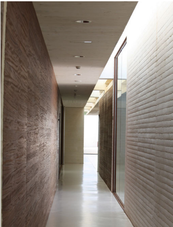
Corridor in the Museum staff wing, on the east side of the central patio. Hand-made casement windows in coreten steel are placed on the inside of the mashrabiyya-like openings.
