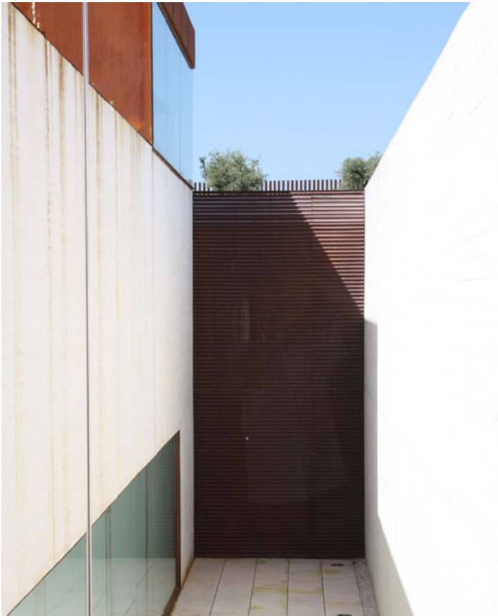
The "work yard" along the office wing, terminated by a massive corten panel.
