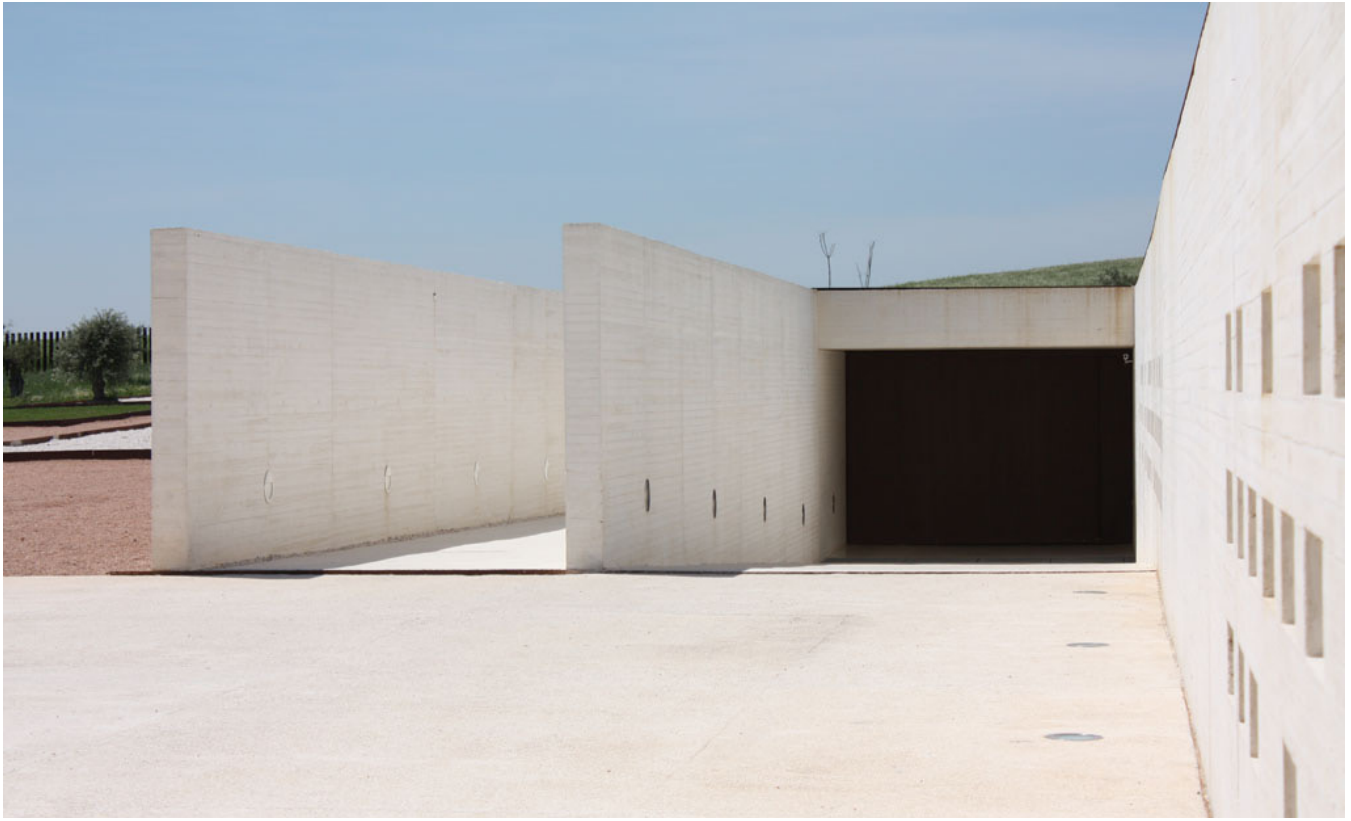
View of entry.
