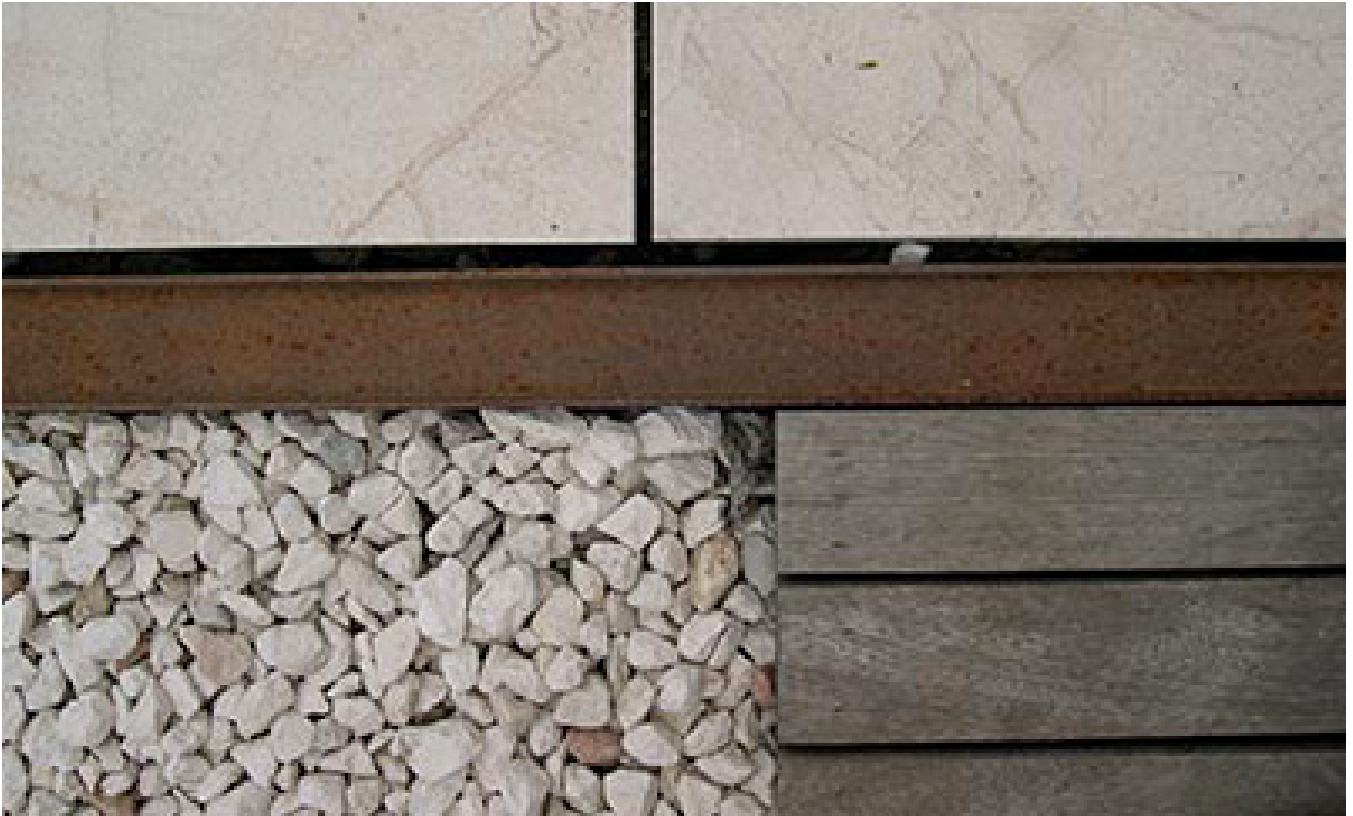
Detail of materials at central patio.
